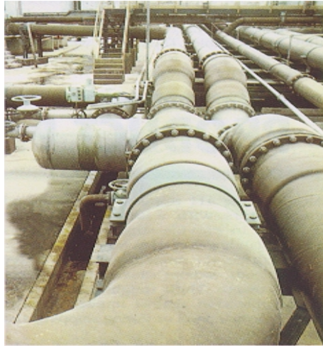
Figure 3. Abrasion Resistant Pipe for Corrosive Slurry
