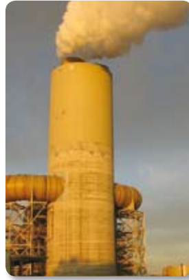
Fig. 2. Chimney with two FRP stack liners in operation in North Carolina.
