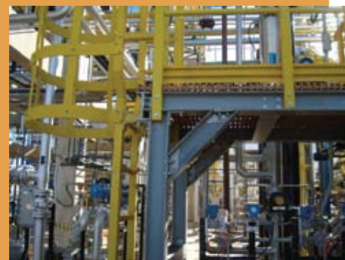
Pultruded gratings, railings and structural members for Petrobras platform
