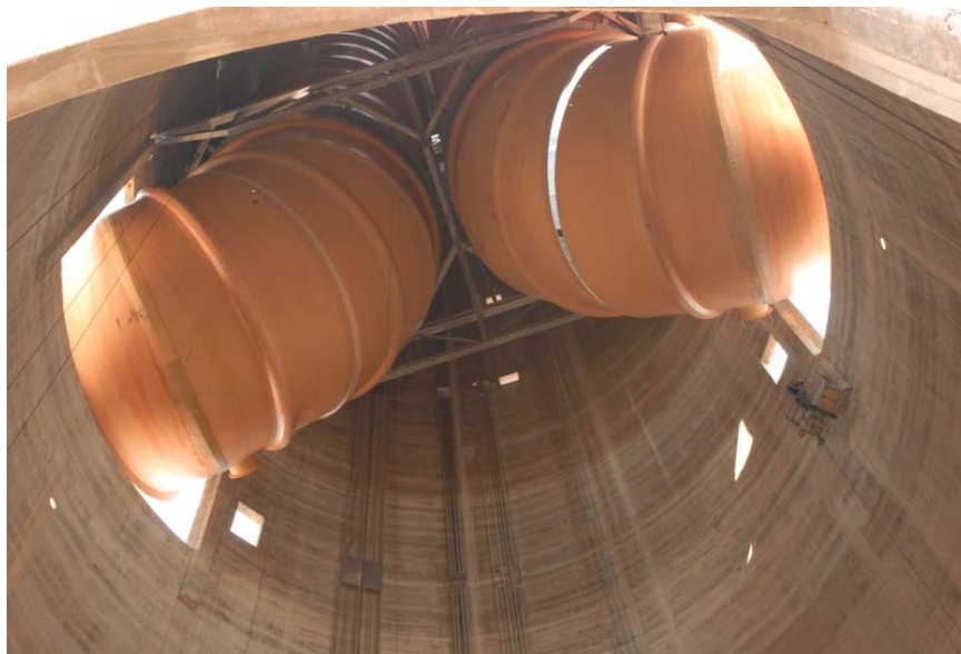
Figure 8. Stack Liner Installation in a Power Plant on the East Coast.
