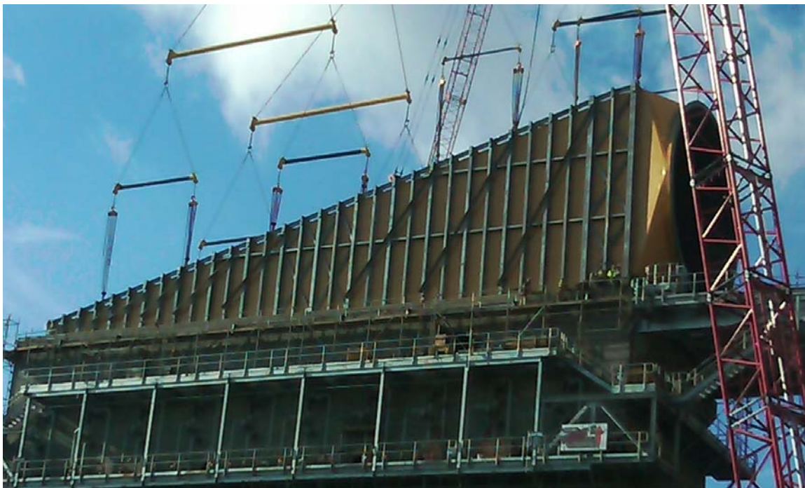
Figure 1. FRP Scrubber Hood Saves Utility $4.2 MM Compared to C-276
