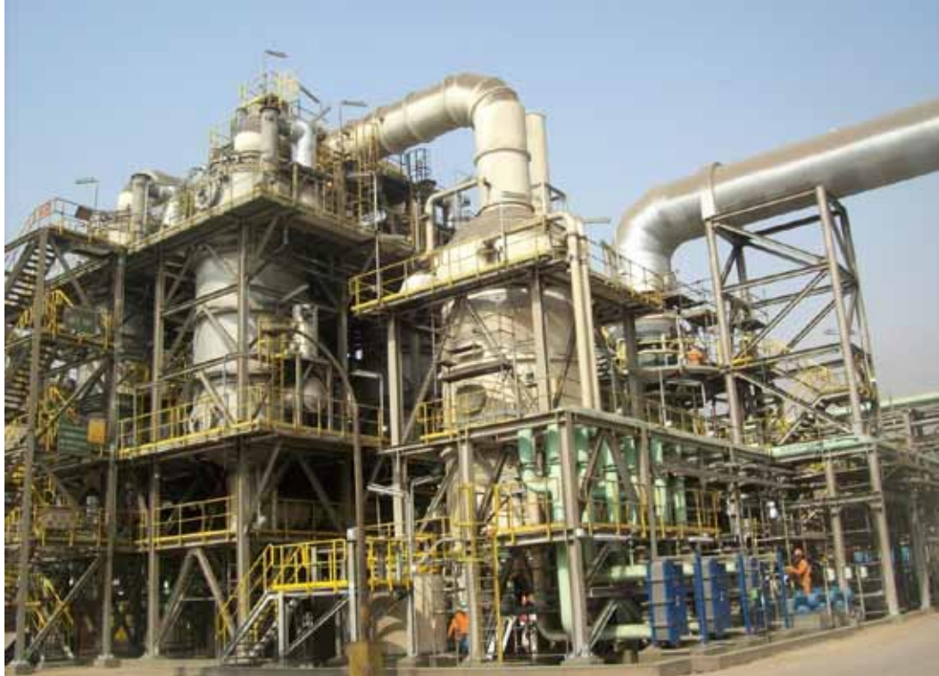
Cajamarquilla Sulfuric Acid Plant Made with Extensive Use of FRP
