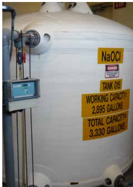
FRP tanks typically last twice as long as HDPE in Hypo service
